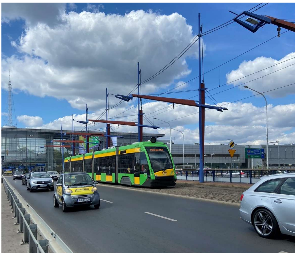
Figure 3-2. Segregated on road Mass Transit corridor (Poznan, Poland)
