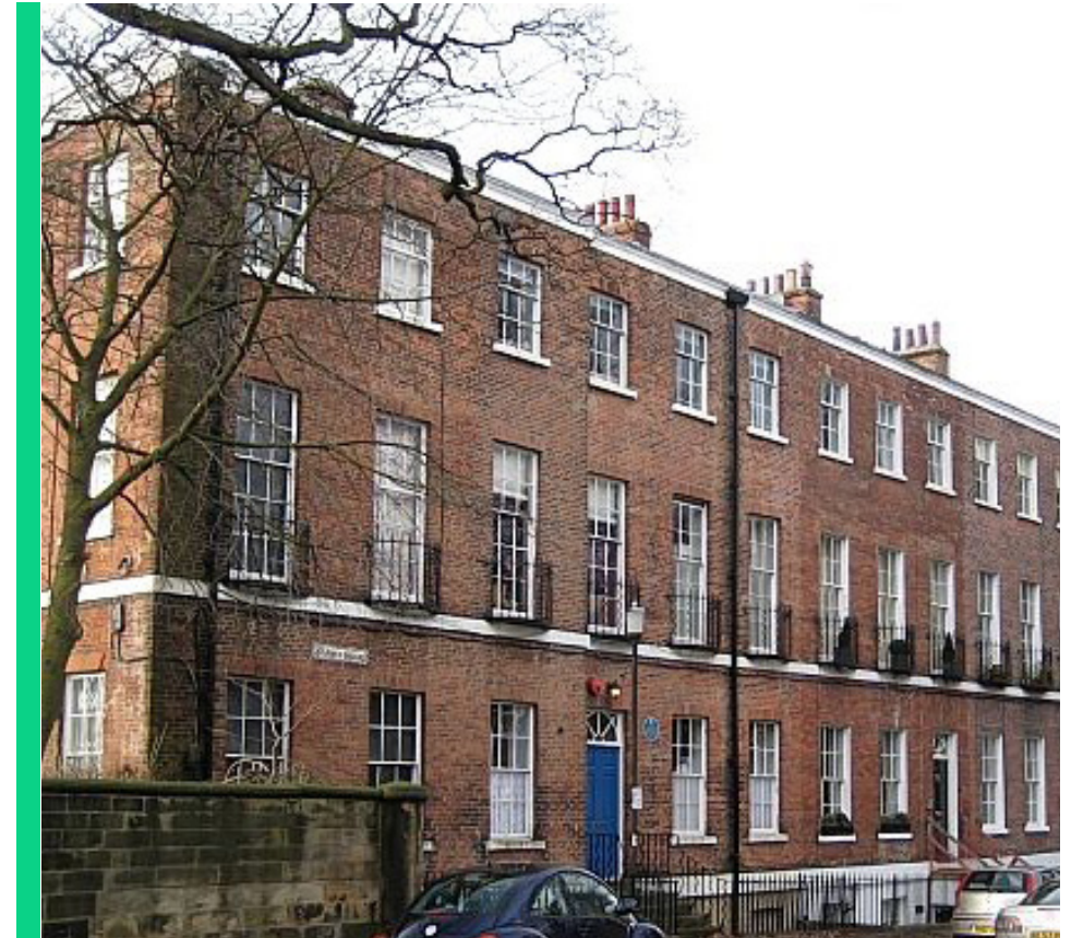
Brick Georgian facade
