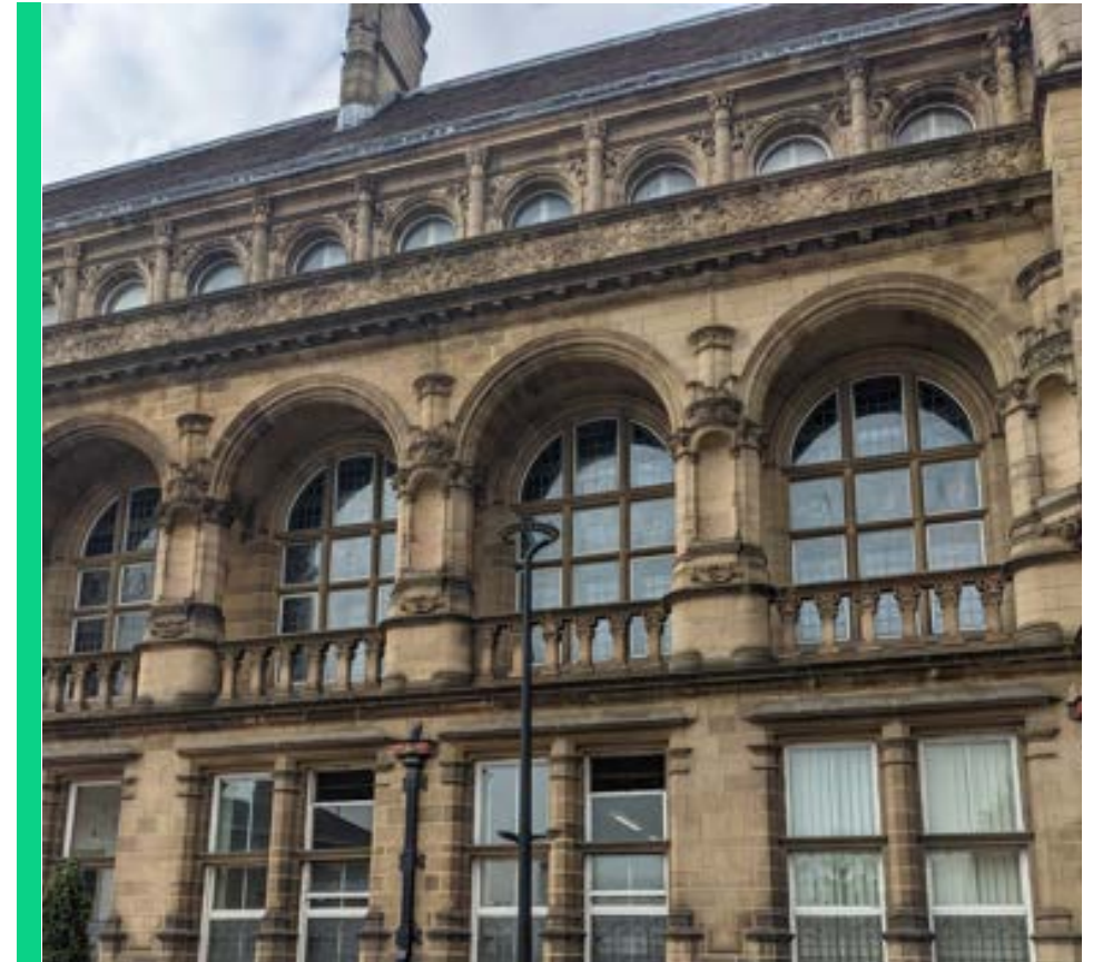
Civic architecture with intricate detail and texture
